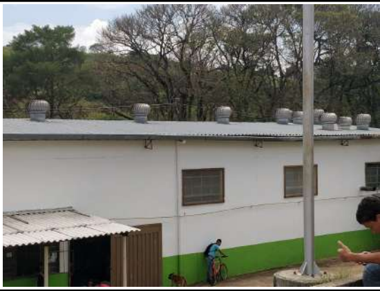
Figure 15: Campus Machado Coffee Roasting Building exhausters.
