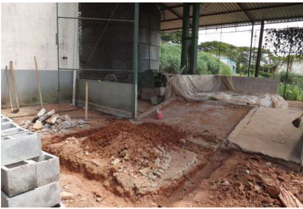
Figure 13: Machado Campus Feed Factory improvements.
