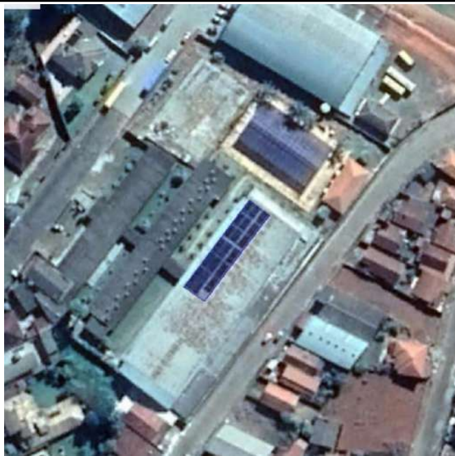
Figure 19. Muzambinho Campus CeCAES Solar water heating system.
