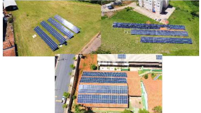
Figure 48: Inconfidentes Campus installation of new photovoltaic panels.
