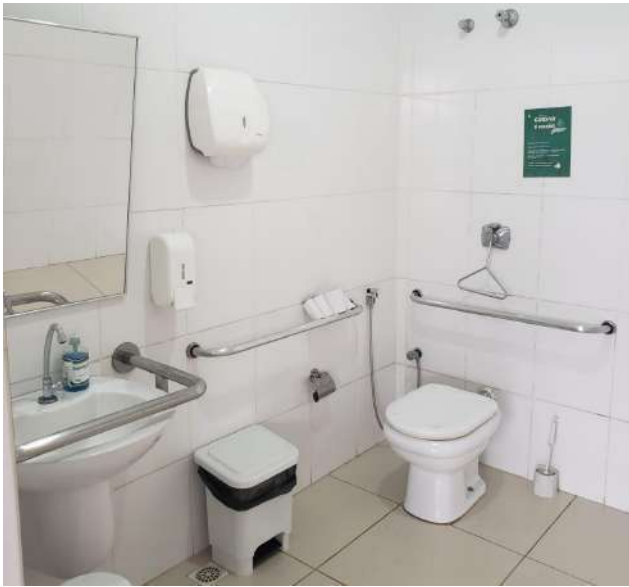
Figure 5: Rectory accessible toilet for people with special needs.
