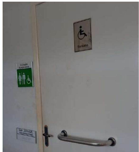
Figure 12: Pouso Alegre Campus accessible toilet for people with special needs.
