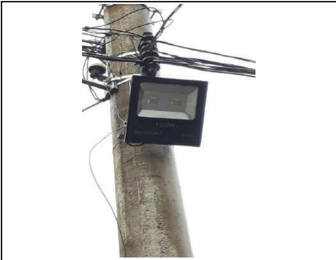
Figure 11: Campus Carmo de Minas high-efficiency luminaires with automatic lighting control – LED lamp post.
