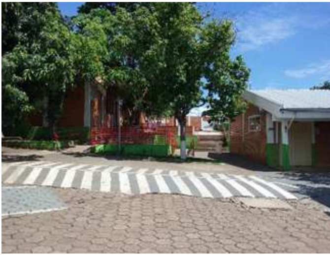
Figure 11: Passos Campus elevated crosswalk.
