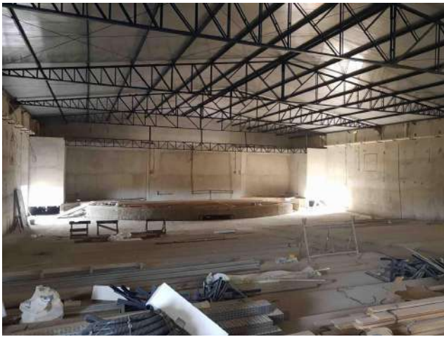
Figure 53: Construction of the Muzambinho Campus Auditorium.
