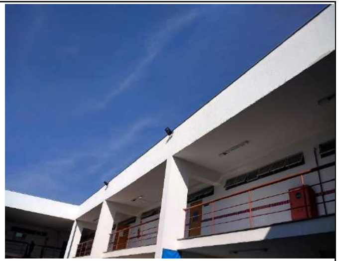
Figure 12: Campus Poços de Caldas high-efficiency luminaires with automatic lighting control – LED spotlights.
