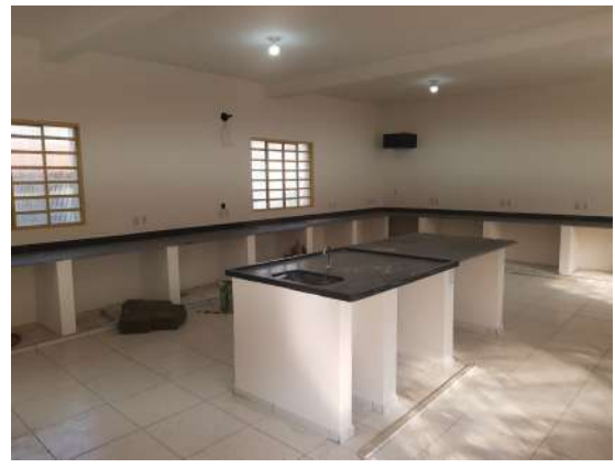
Figure 18: Machado Campus renovation of the Zoology Laboratory.
