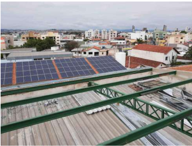
Figure 27: Rectory roof renovation.
