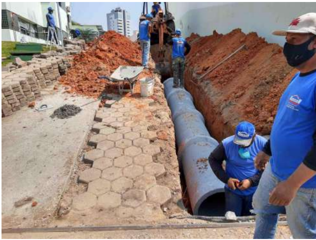
Figure 29: Rectory renovation of the drainage system.
