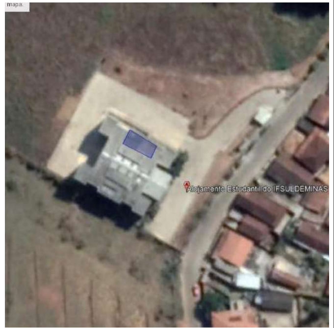
Figure 16. Inconfidentes Campus Solar water heating system.
