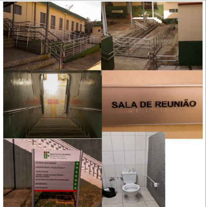
Figure 14: Inconfidentes Campus tactile paving, ramp, handrails, Braille nameplates and bathroom for people with disabilities.
