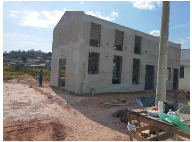
Figure 54: Construction of the Chemical Warehouse at the Poços de Caldas Campus.
