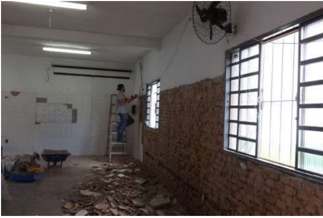
Figure 17: Machado Campus renovation of the Zoology Laboratory.
