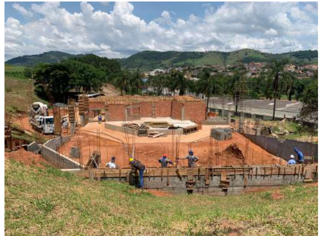
Figure 50: Construction of the Inconfidentes Campus Auditorium.
