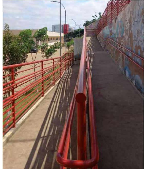
Figure 10: Pouso Alegre Campus ramp and handrails.
