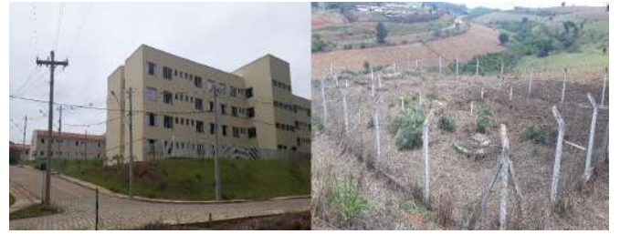
Figure 6: Muzambinho Campus waste treatment.
