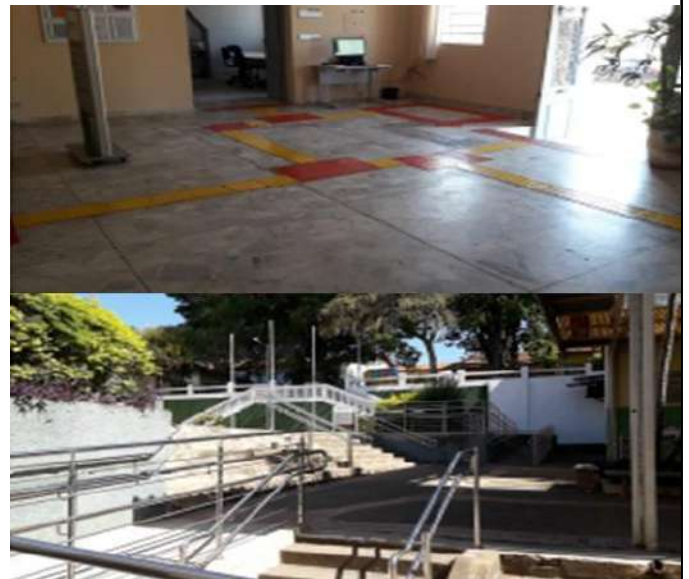
Figure 8: Inconfidentes Campus tactile paving, ramp and handrails.
