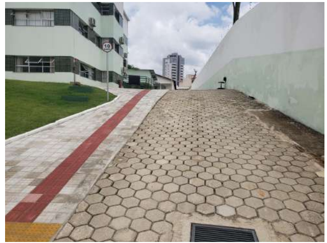
Figure 30: Rectory renovation of the drainage system.
