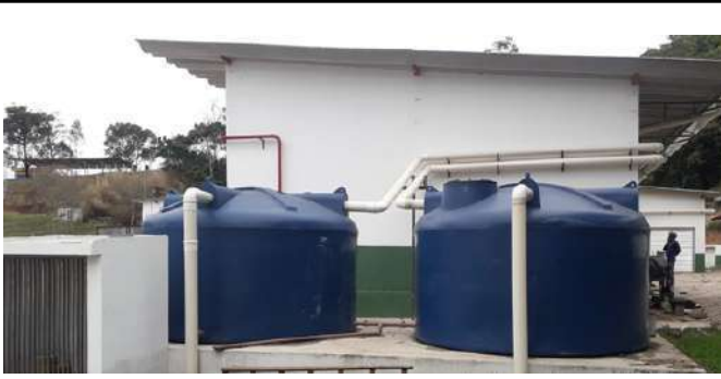
Figure 13: Carmo de Minas Campus rainwater reservoir tanks.
