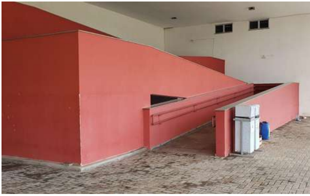
Figure 13: Poços de Caldas Campus ramp and handrails.
