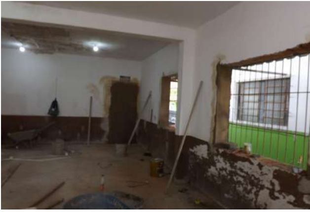
Figure 5: Machado Campus renovation of the Nursing Laboratory.
