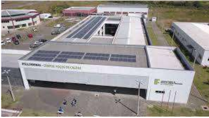
Figure 5: Campus Poços de Caldas solar power plant.
