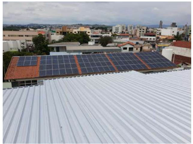
Figure 28: Rectory roof renovation.
