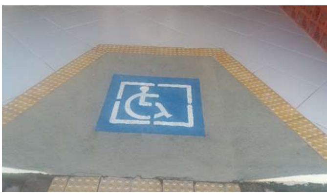
Figure 1: Rectory curb ramp.
