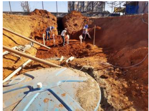
Figure 10: Machado Campus construction of Sewage Treatment Network in Center of Excellence of Coffee.
