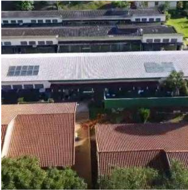
Figure 15. Inconfidentes Campus Solar water heating system.
