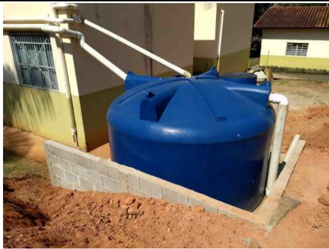
Figure 5: Inconfidentes Campus rainwater reservoir tank.
