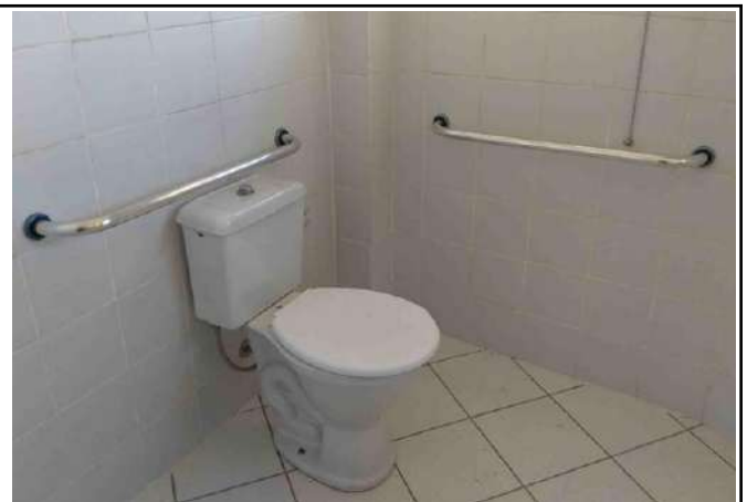
Figure 2: Rectory toilet water box flush.
