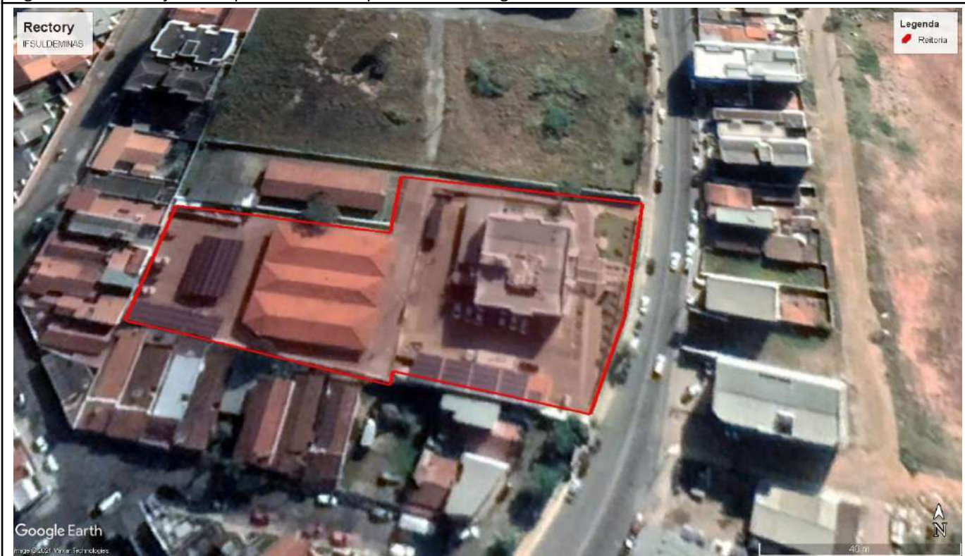
Figure 11: IFSULDEMINAS Rectory. Source: Google Earth.
