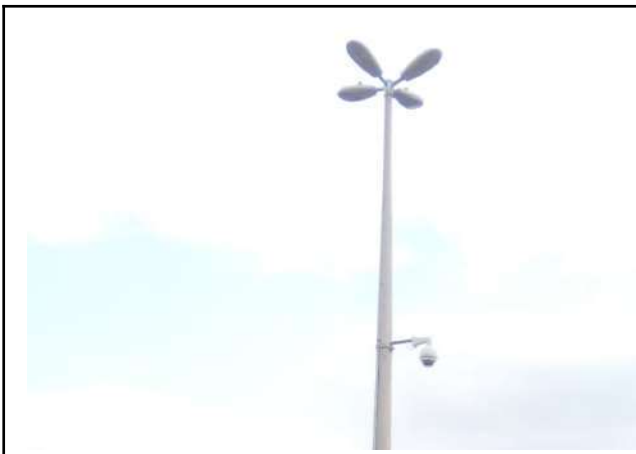
Figure 1: Machado Campus 360° monitoring camera.
