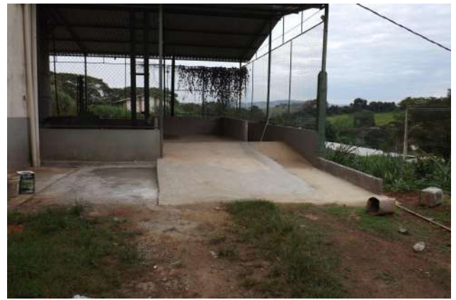
Figure 14: Machado Campus Feed Factory improvements.
