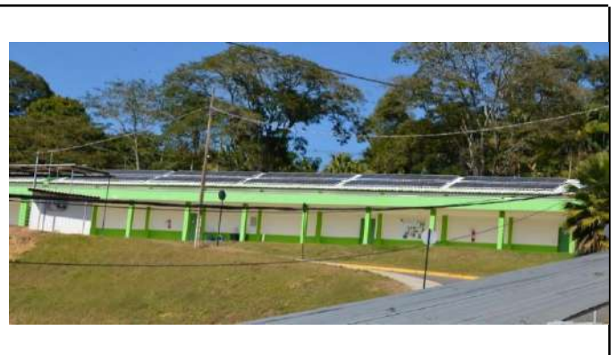
Figure 2: Campus Machado solar power plant.
