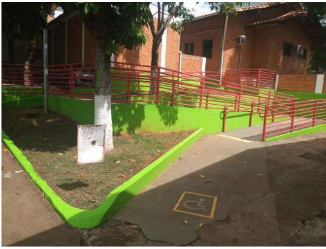
Figure 17: Passos Campus ramp and handrails.
