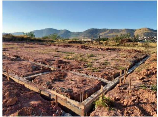
Figure 36: Inconfidentes Campus construction of a new teaching block for classrooms.
