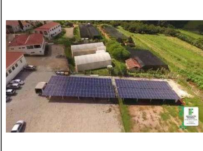
Figure 3: Campus Muzambinho solar power plant.
