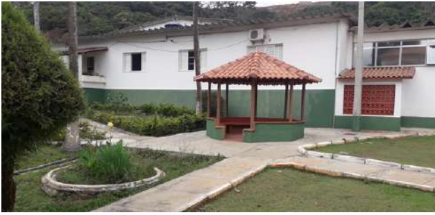
Figure 23: Carmo de Minas Campus Bandstand reformed with its original architecture.
