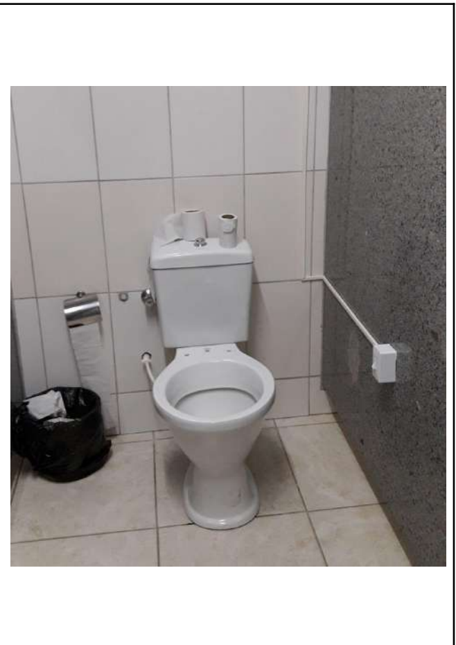
Figure 12: Inconfidentes Campus panic button on the toilet for people with special needs.
