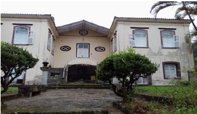
Figure 25: Carmo de Minas Campus old mansion before renovation.
