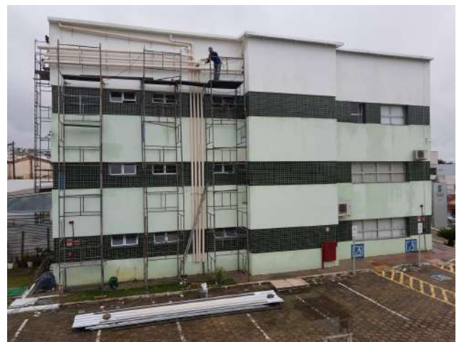
Figure 32: Rectory renovation of the rainwater collection system.
