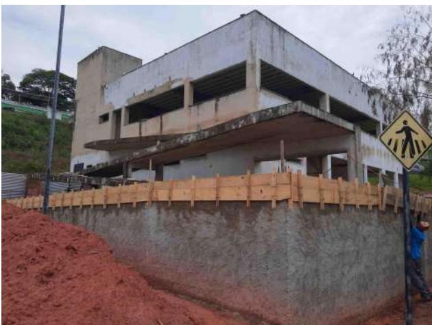
Figure 51: Construction of the Machado Campus Innovation Hub.
