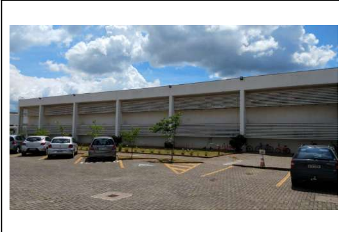
Figure 15: Campus Poços de Caldas shielding adjustment and solar control – Brise-soleil at classroom building.
