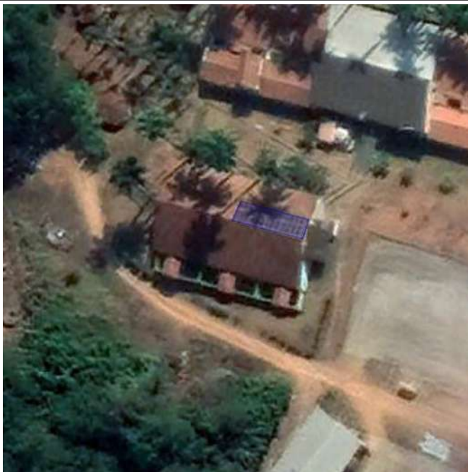
Figure 17. Machado Campus Solar water heating system.
