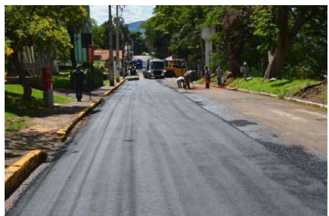
Figure 4: Machado Campus street paving refurbishment.
